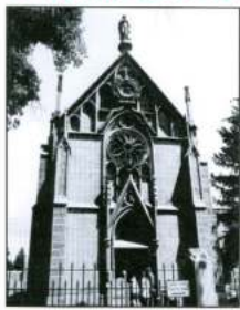
Loretto and the Miraculous Staircase
